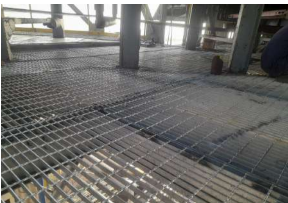
GRATING INSTALLATION AND FENDER STRUCTURE REPAIR WORK AT ADANI PORT
